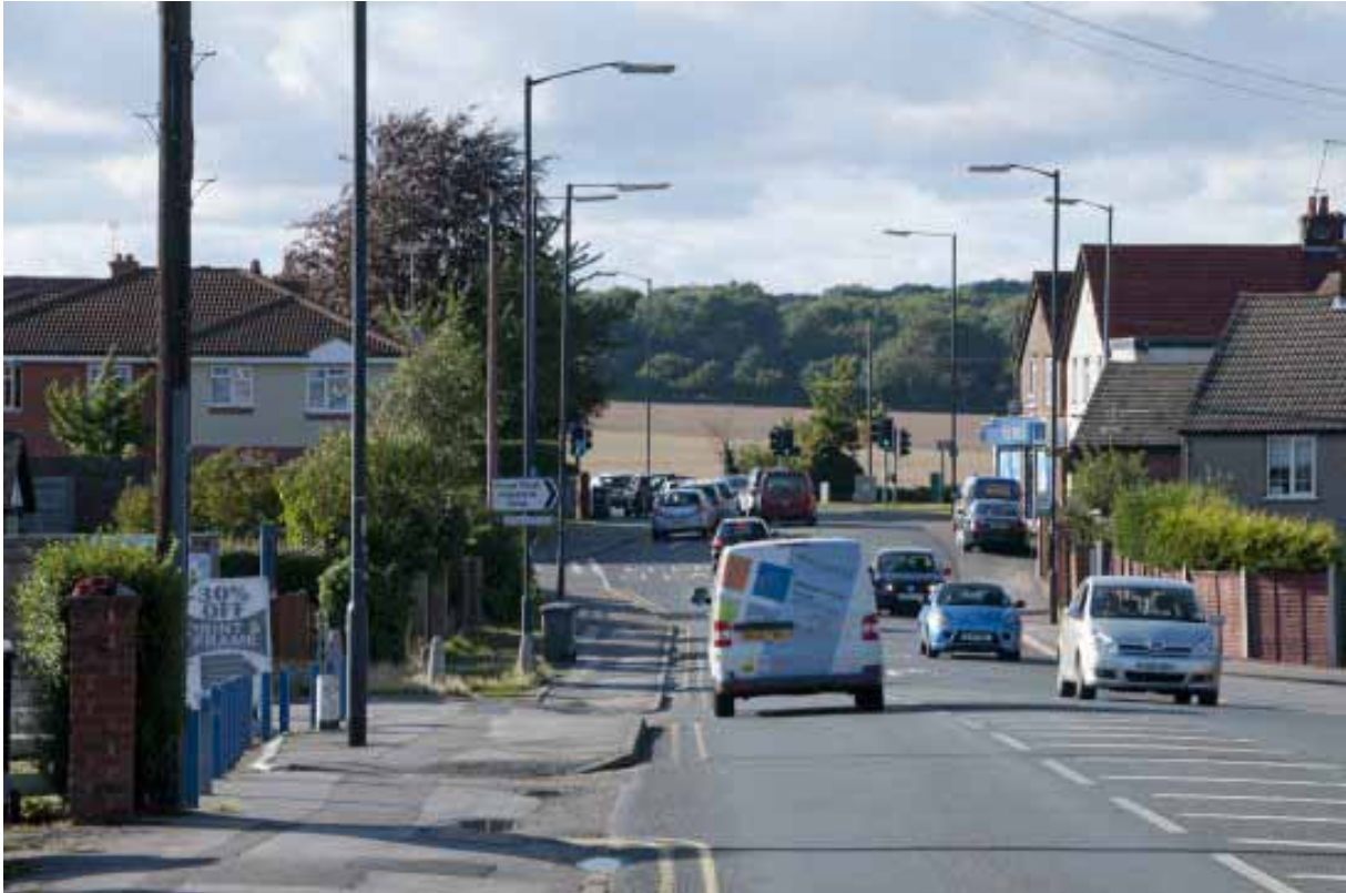
At the junction of Linden Avenue and Gringer Hill, looking east the land drops away giving a view in winter across to the far side of the Thames valley, with glimpses of the distant gravel workings which may have been a source of local gravel drives and pebbledash. To the north can be seen the arrayed frontages of houses on the west side of Furze Platt Road, mixed with the greenery of trees in their front gardens.
